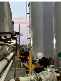
Kig Iccp Testing Station Installation
